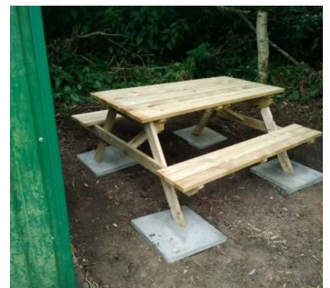
New bench in clearing created by cutting back nettles and sitting on spare slabs to prevent the table soaking up damp.
